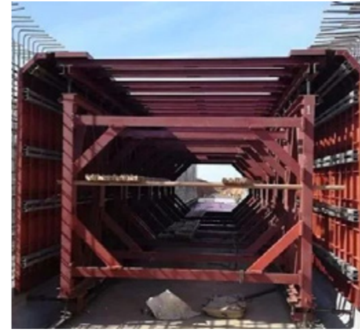
Pipe Gallery Steel Formwork Support System 管廊钢模支撑体系
