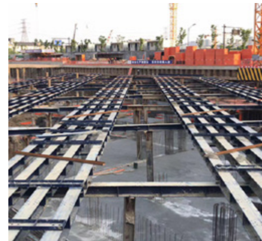
Steel Support System for Foundation Pit 基坑钢支撑体系
