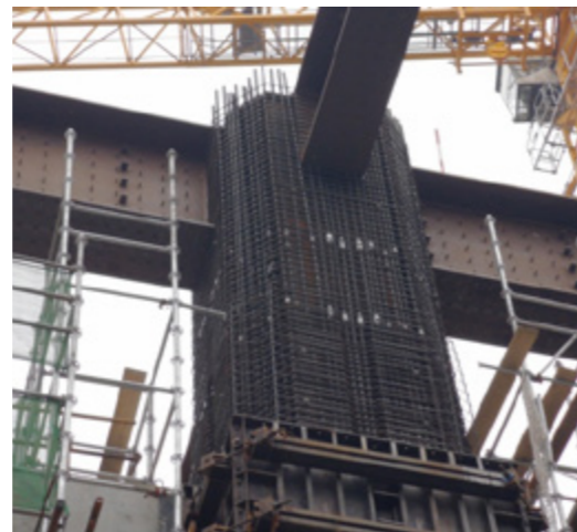
Heavy Steel Ultra-High-Rise Stiffness Columns and Beams 重钢超高层劲性柱梁
