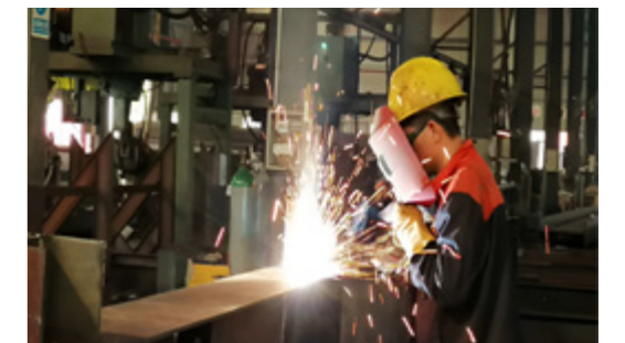
Assembly, Welding 组装、焊接
