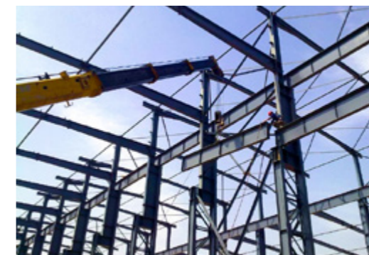
Light Steel Factory Building 轻钢厂房
