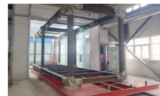
Rust Removal, Painting 除锈、喷漆
