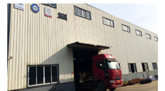
Loading and Transportation to the Construction Site 装车运送至工地
