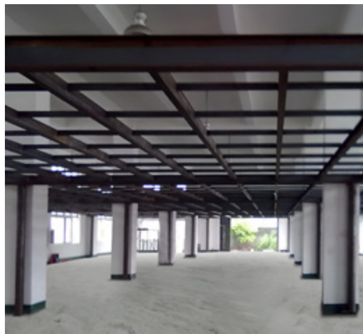
Steel Structure Mezzanine 钢结构夹层
